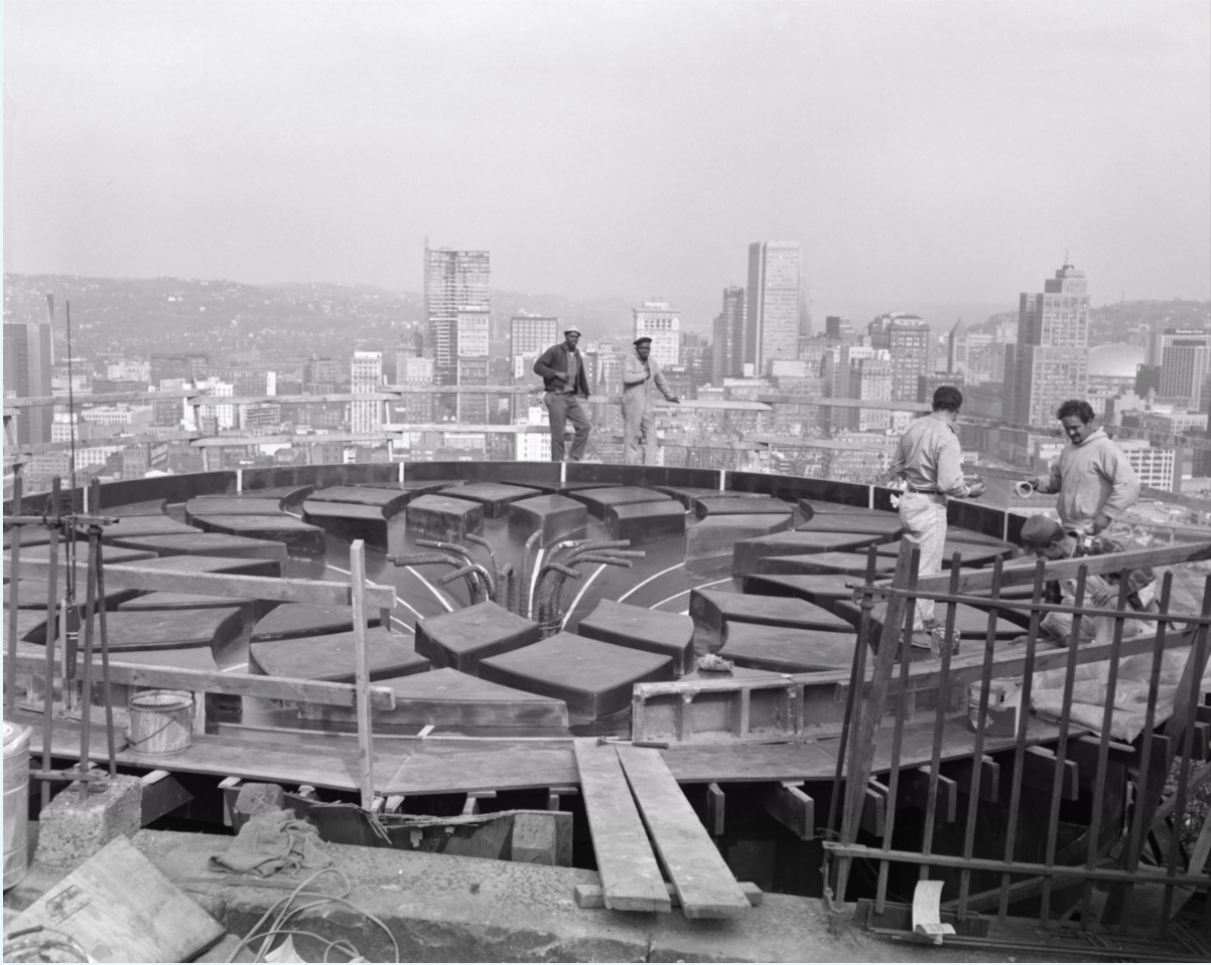
Overlook construction, October, 1967. Pittsburgh City Photographer Collection, 1901-2000, University of Pittsburgh.
