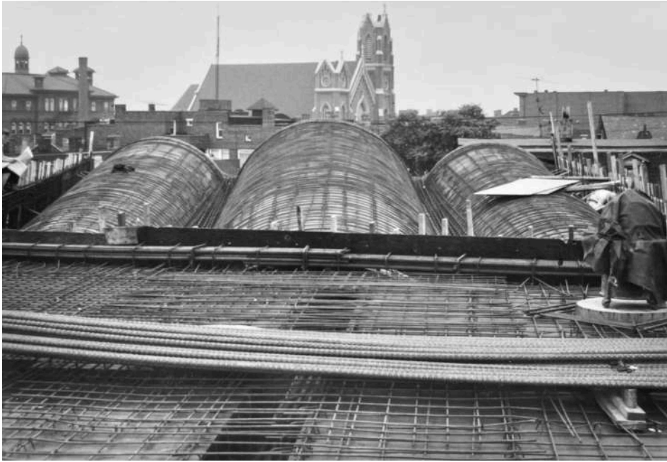
Formwork and rebar installation are completed on August 26, 1960.
