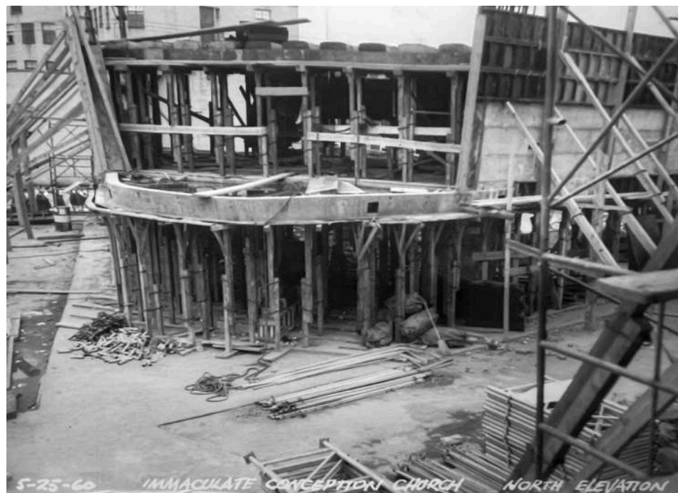
Choir loft formwork, May 25, 1960.
