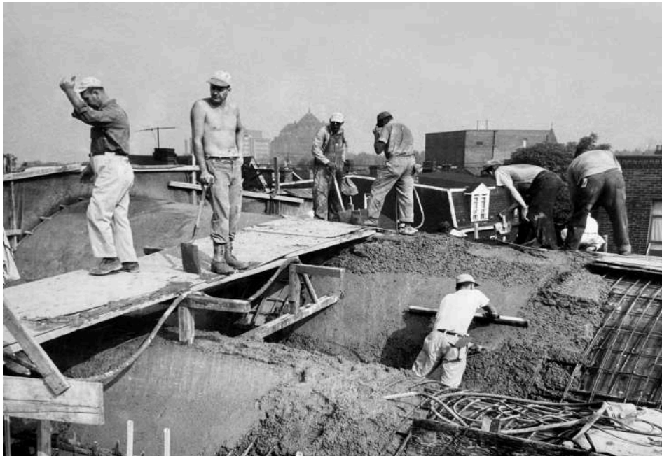
The concrete pour began on September 5th, 1960
