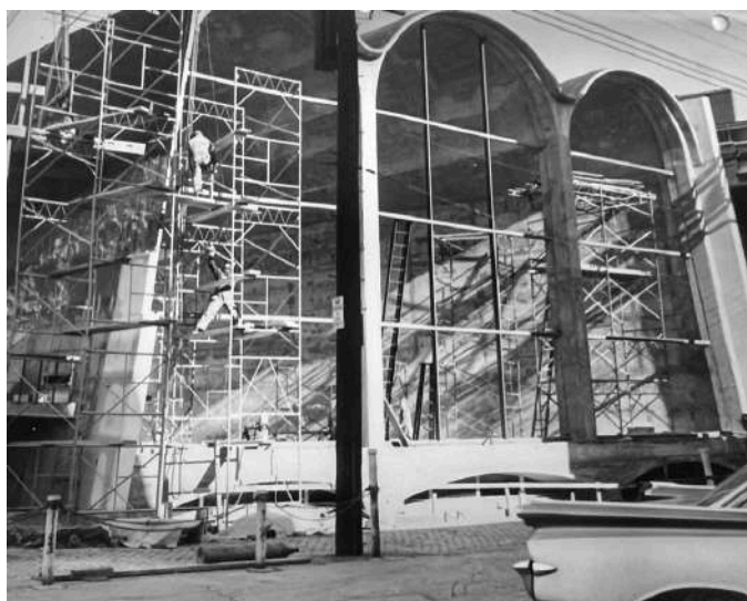
Stained glass framework is installed in the south nave.
