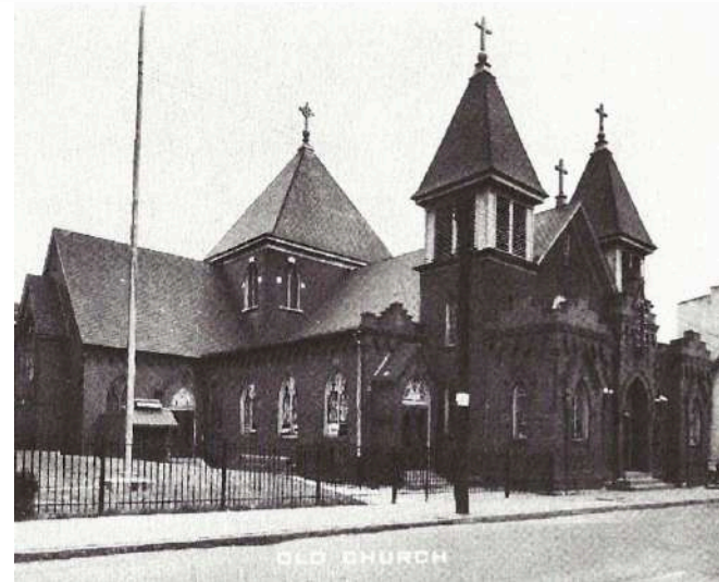
The 1906 Immaculate Conception Church. Structural damage from a fire would eventually necessitate a new church.
