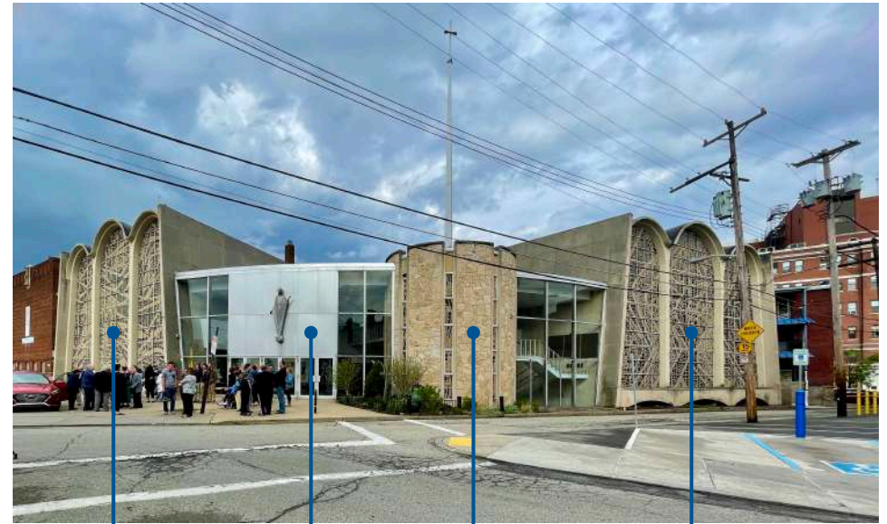
West Facade (West Nave)
